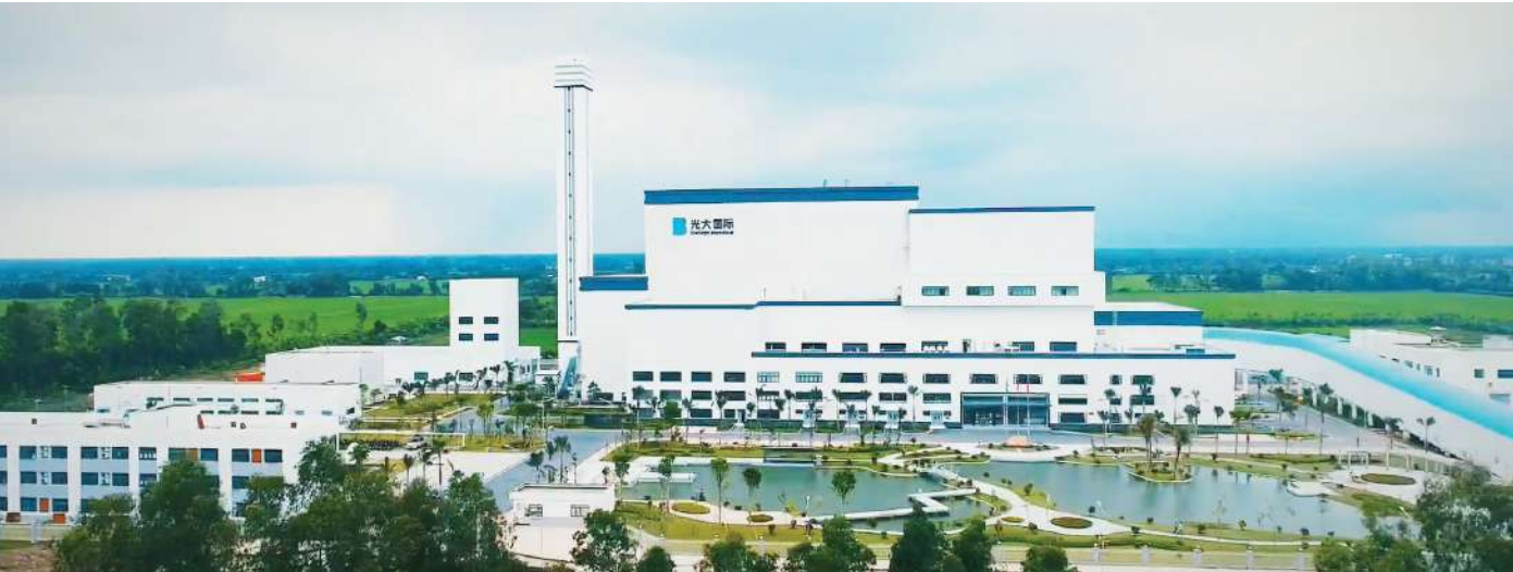
Can Tho Thermal Power Plant
